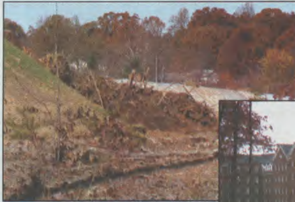
Above is a portion of the area recently stripped of trees. At right is the area where the protested trees fell. Photos by Mike Nuckles.
